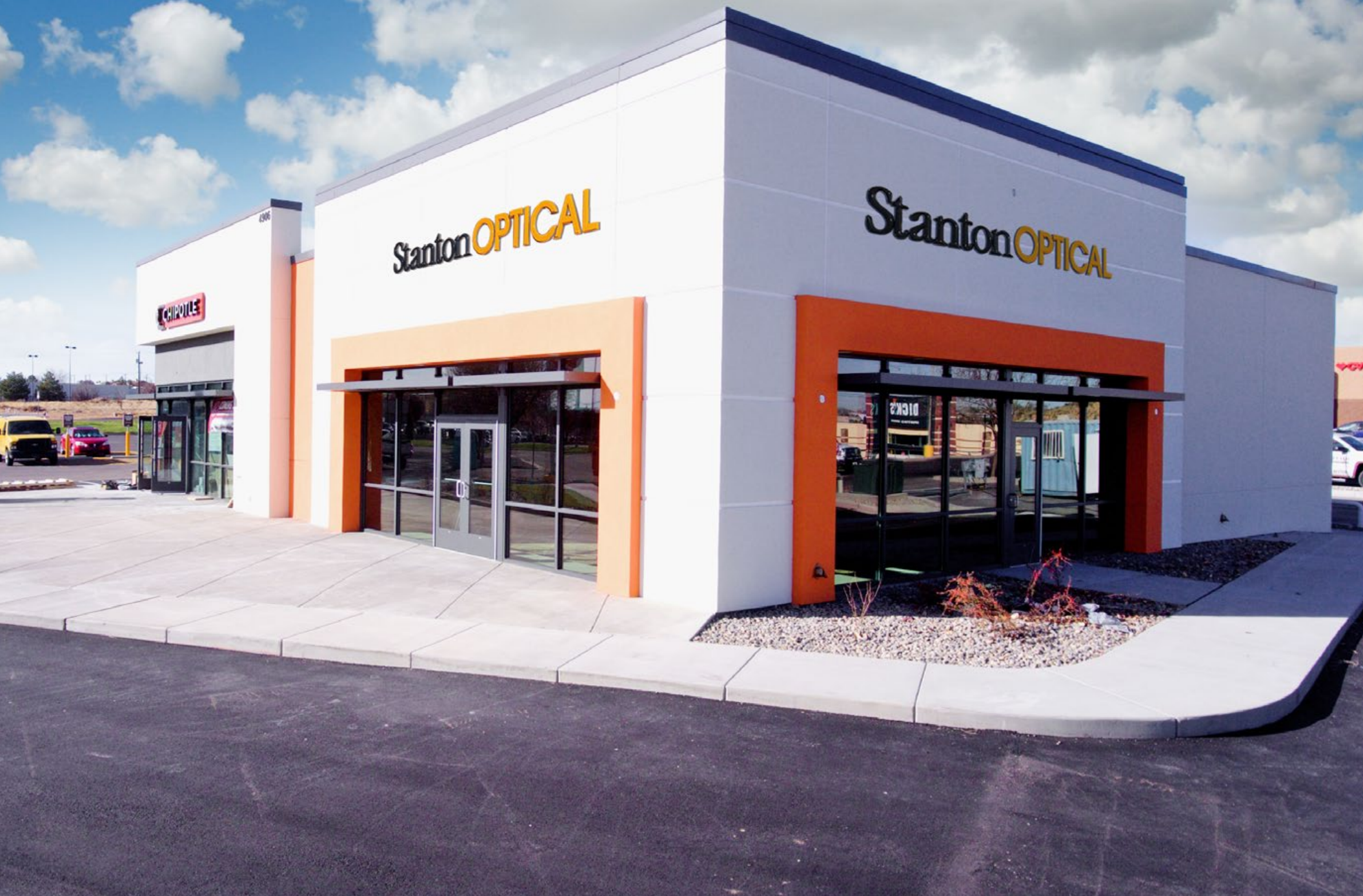
Actual Site (Under Construction / Photos Taken Nov. 2017)
